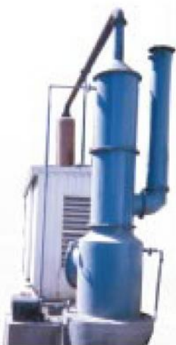
320 KVA automatic DG set with FGDC Scrubber installed at Hutchison Max, Mumbai
