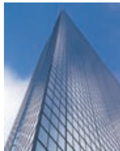
HVAC / Building management
